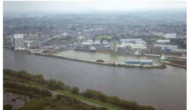
Photo 37 - Limerick Docks as a working Port
