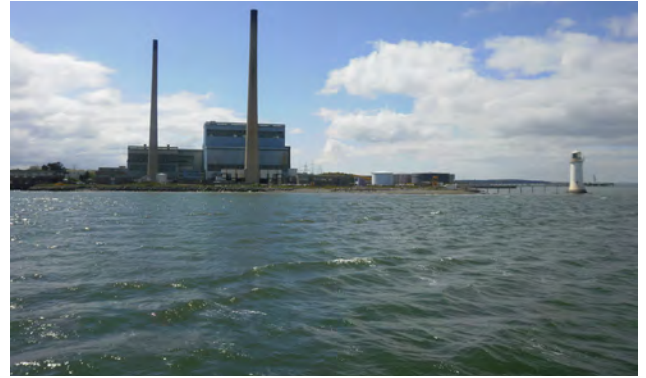
Photo 33 - Tarbert Power Station, Tarbert
