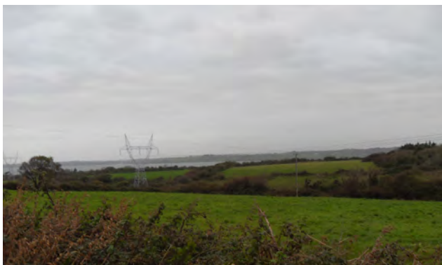
Photo 12 - Important grid infrastructure at Labasheeda
