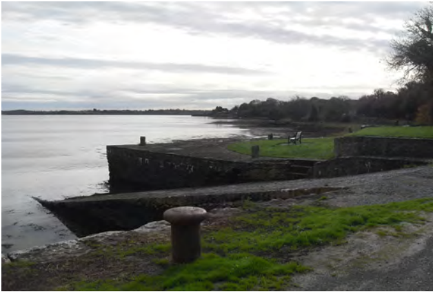
Photo 51 Improvements to existing facilities & infrastructure
