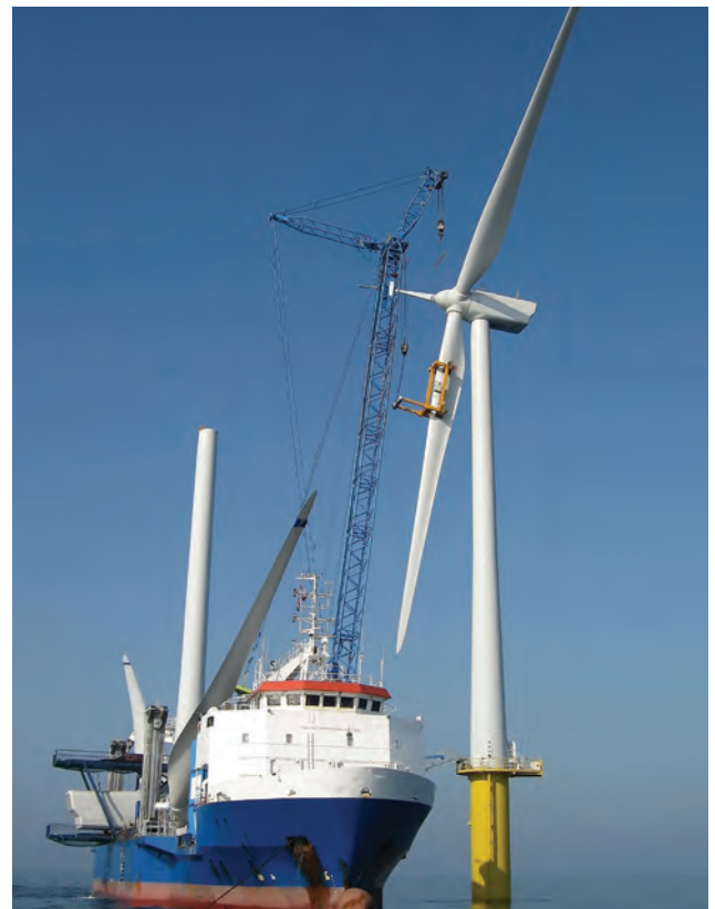
Photo 46: Construction of an offshore wind farm
