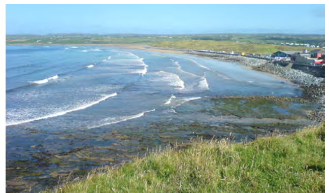
Photo 60 Coastal Protection along Coast Road, Lahinch
