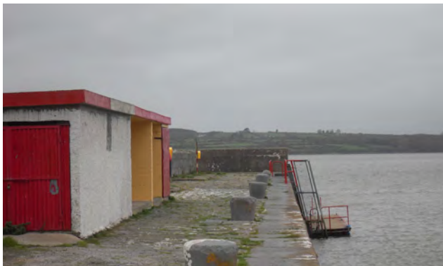
Photo 11 - Glin Pier, Glin, Co Limerick
