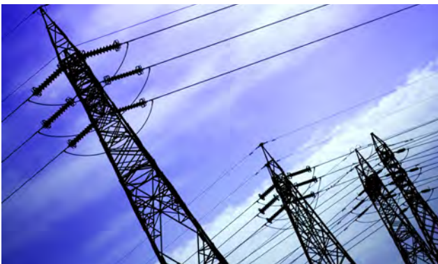
Photo 43 - Upgrading of Electricity Infrastructure is ongoing
