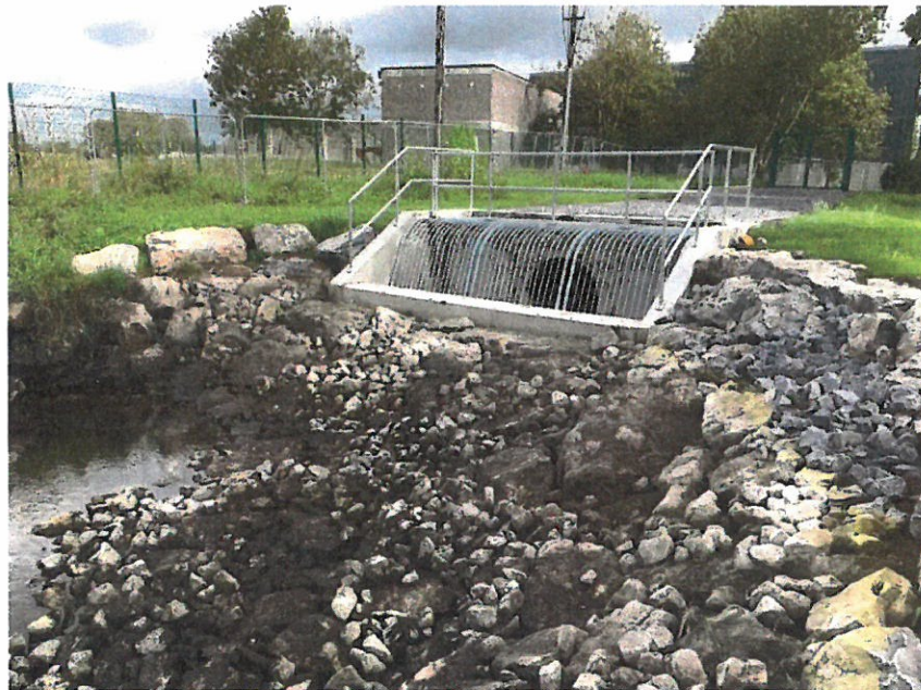
Plate 1 Flood Overflow diversion at the St. Flannans Swallow Holes with inlet screen and weir photo taken during winter flows and low flow during spring period the existing swallow hole is the pooled water to the near left of the bottom photo.
