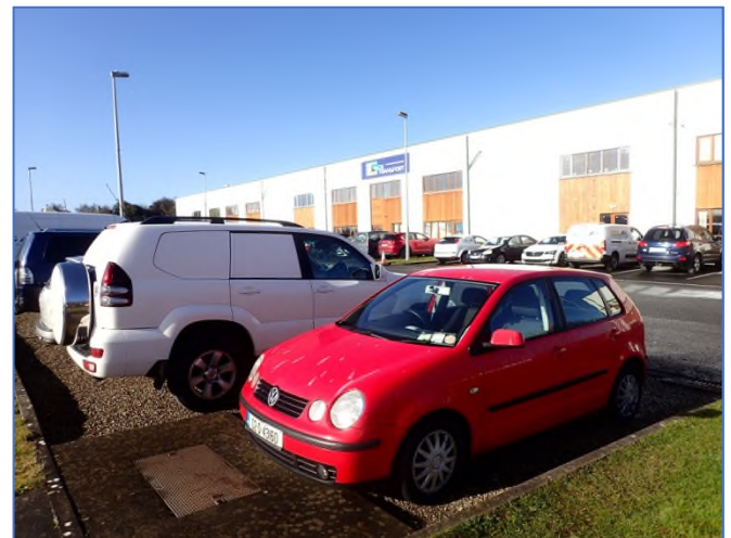
Fig 4 Line of existing industrial units at the western end of the park
