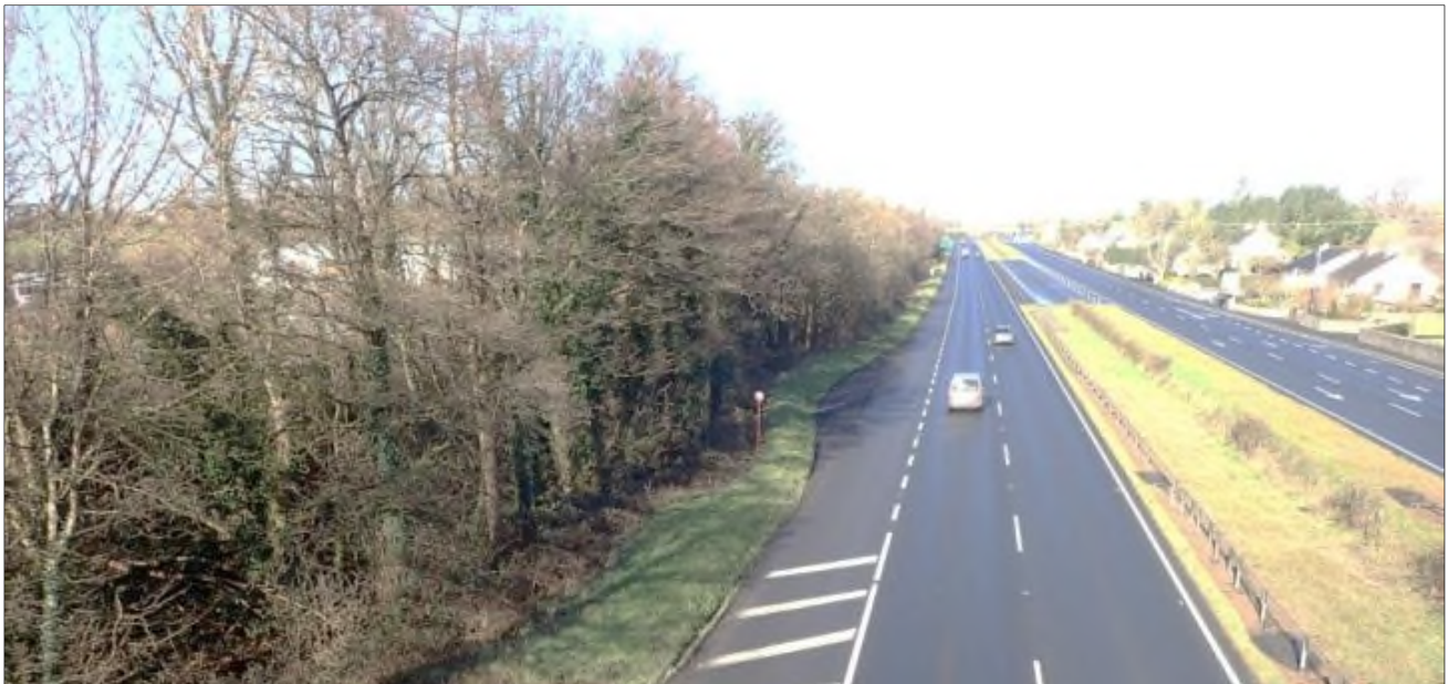
Fig 6 The N18 and industrial park viewed from bridge over the N18. The park is barely visible from the N18 or R462
