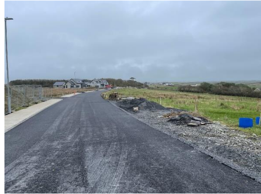
Photograph 4 Showing the Upgraded Road
