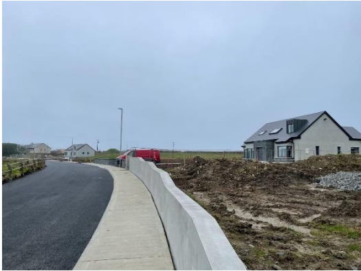
Photograph 3 Showing the Footpath Provision Linking the Site and Public Road
