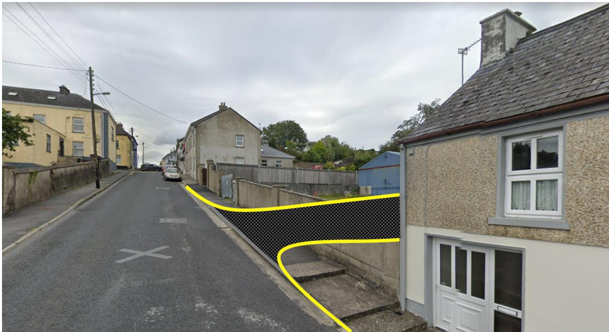
Image with access road
