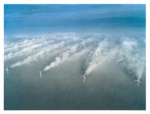
Above shows the impact that "Near" and "Far" wake turbulence will have downwind of wind turbines.
