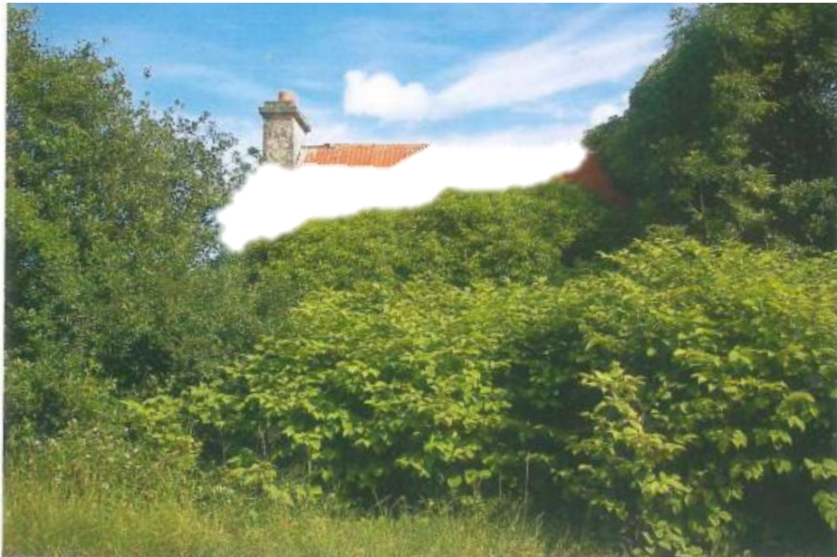
Site A – Derelict Cottage
