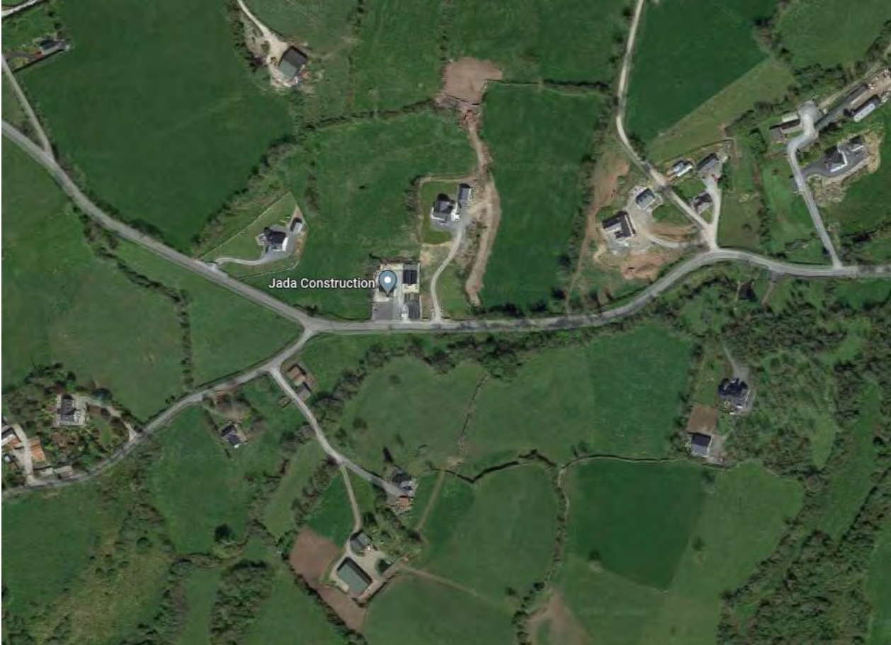
Figure 4 - Aerial Image of Builders Compound and Storage Yard at Caherbannagh, Fountain, Ennis.
