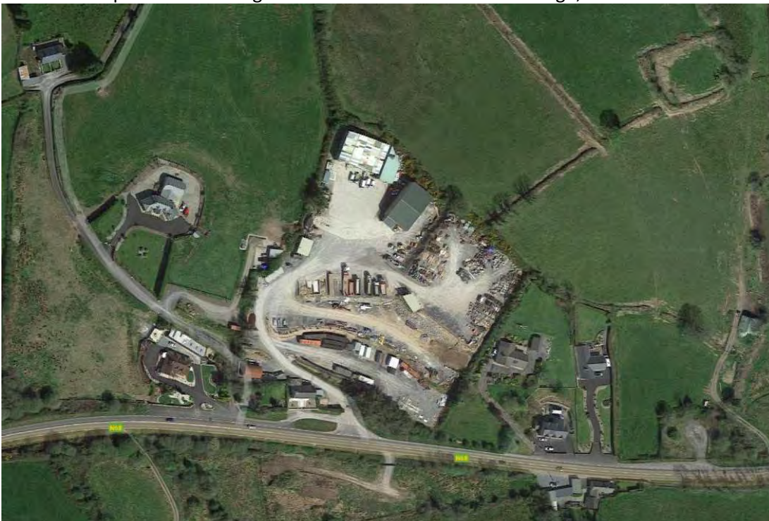
Figure 3 – Aerial Image of Builders Compound and Storage Yard at Darragh, Ennis.
