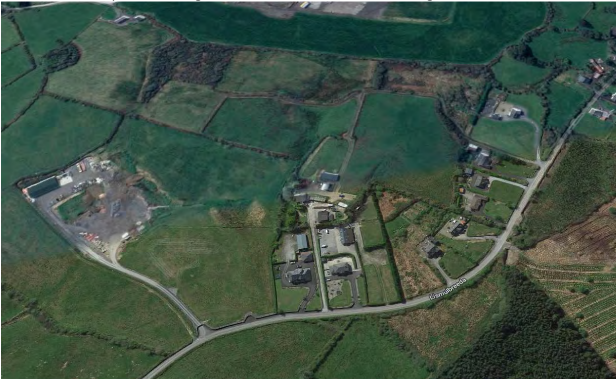
Figure 6 – Aerial Image of Builders Storage Yard and Shed at Lismulbreda, Darragh.
