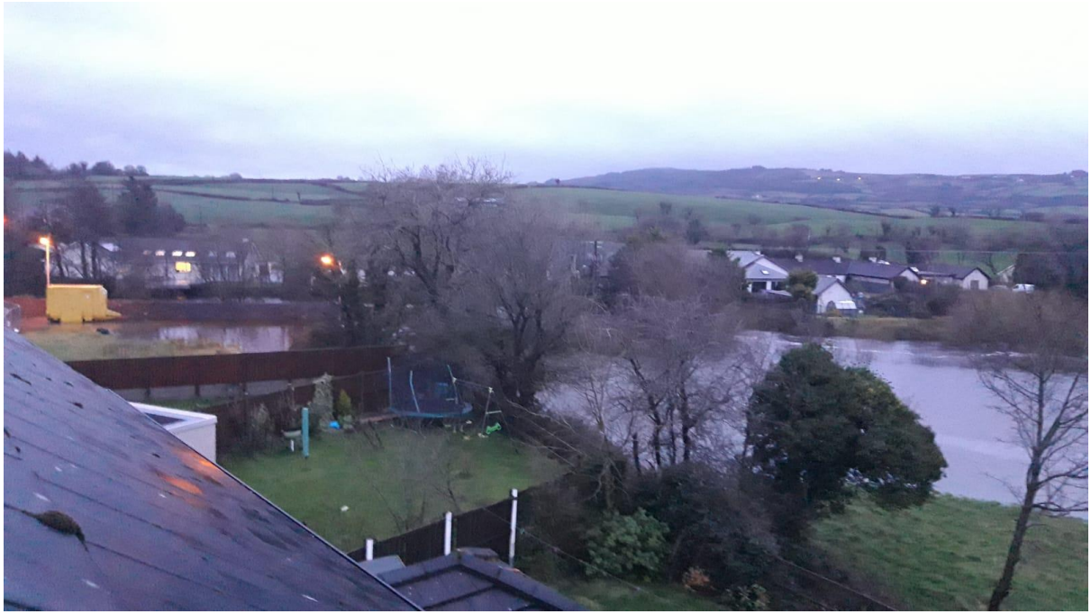
Plate 10 Pumps placed by the council end of 2009/start of 2010
