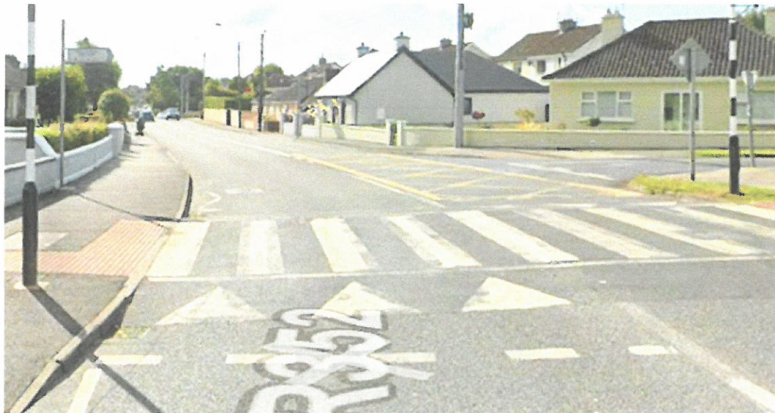
Zebra crossing on Tulla Road and signage for route through to Gort Road
