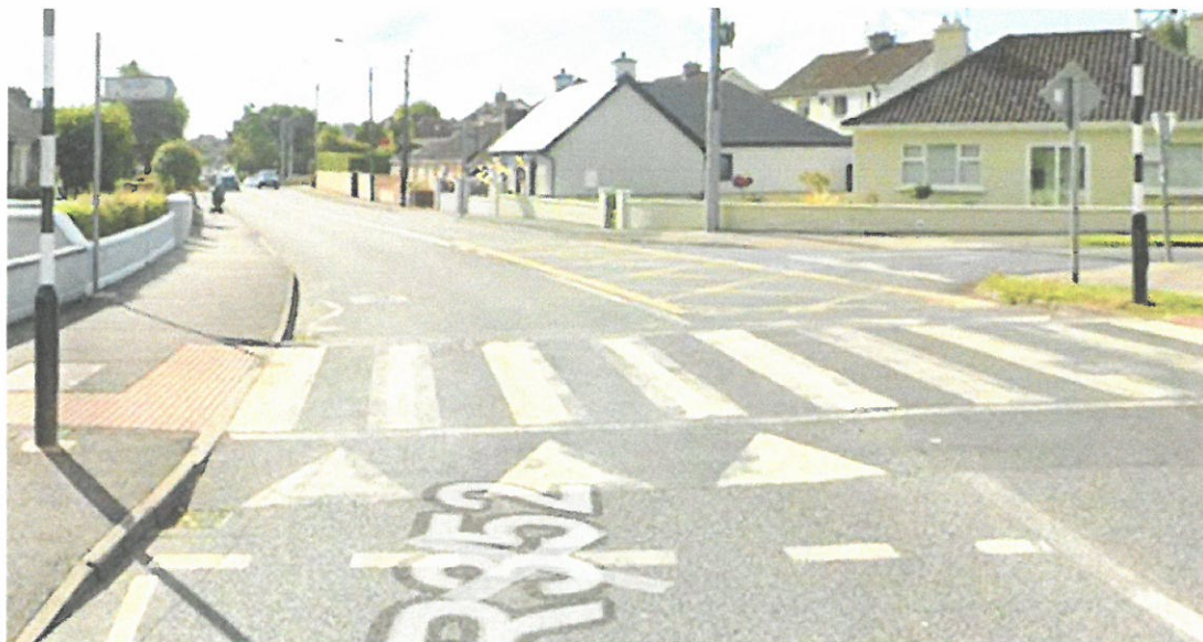
Zebra crossing on Tulla Road and signage for route through to Gort Road
